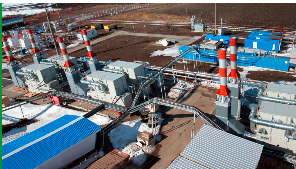
Six OP16 turbines installed at a TNK-BP oil field in Russia
