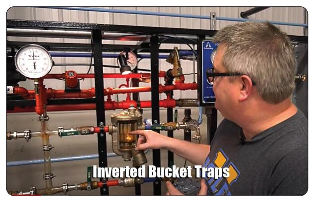
As the bucket rises, it closes a valve that seals off the outgoing condensate line. By doing this, it prevents any steam from escaping.
